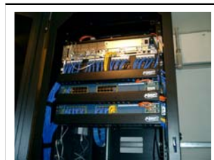
New EEC Network Installation
