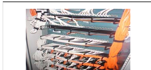
New LAN Installation
