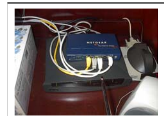
Old EEC Network Installation
