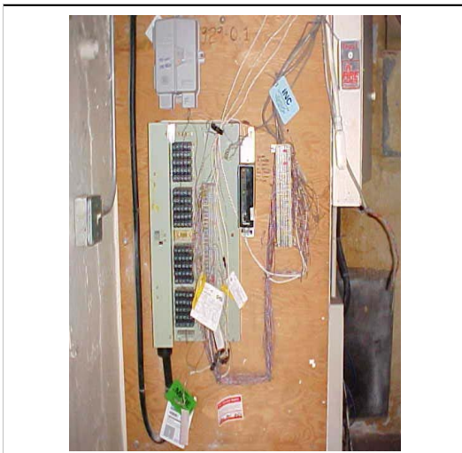
Existing Telephone Wiring Termination Installation
