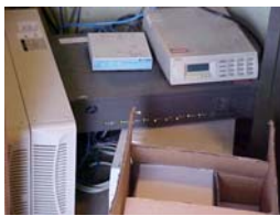
Old Router Technology
